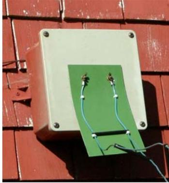
Figure 8 – Transmitter end. Inside the PVC box are threaded ¼” steel rods in PVC pipe going through the wall to the tuner.
